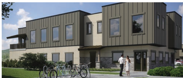
LINCOLN STATION - READY FOR OCCUPANCY 670 W BITNER ROAD • PARK CITY, UTAH 84060 COMMERCIAL LEASE - $25/SF/YR
