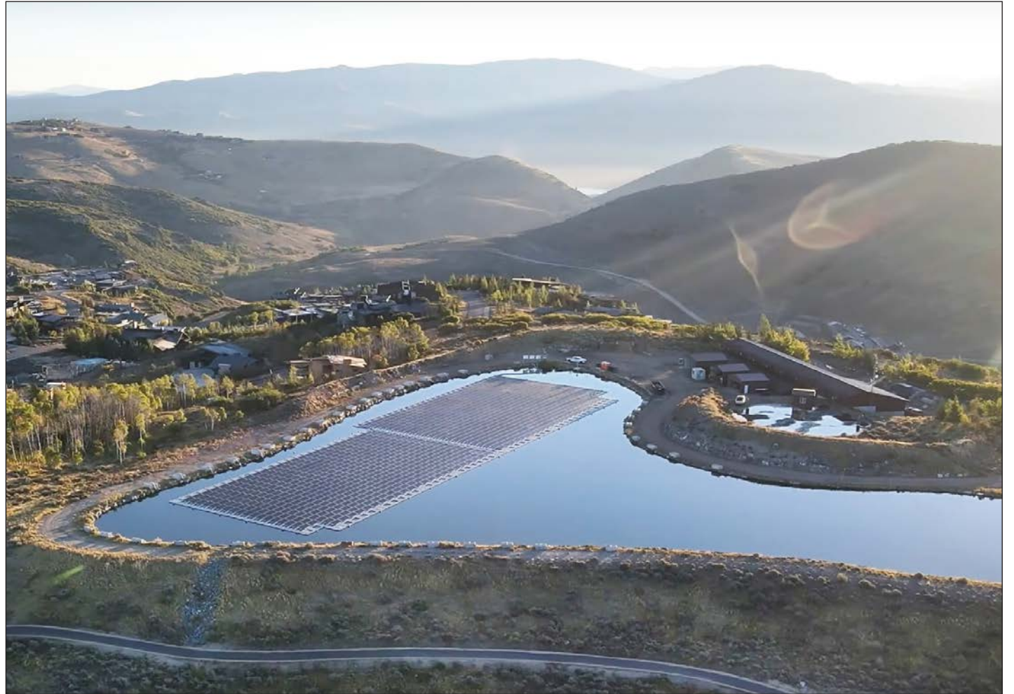
D3Energy, a Florida-based renewable energy company, has begun operation of Utah's first floating solar array. The 600-kilowatt system, deployed on the surface of the collection pond at Mountain Regional Water's Signal Hill Water Treatment Plant near Park City, will supply the bulk of the power to operate the facility. The project uses a Hydrelia floating system manufactured by Ciel & Terre in Petaluma, California.
