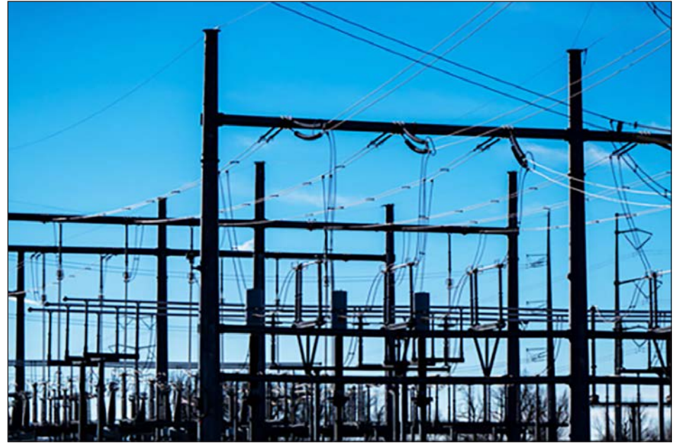
Power transmission lines near the Lake Side natural gas power plant in Vineyard. (Photo by Spenser Heaps for Utah News Dispatch)
