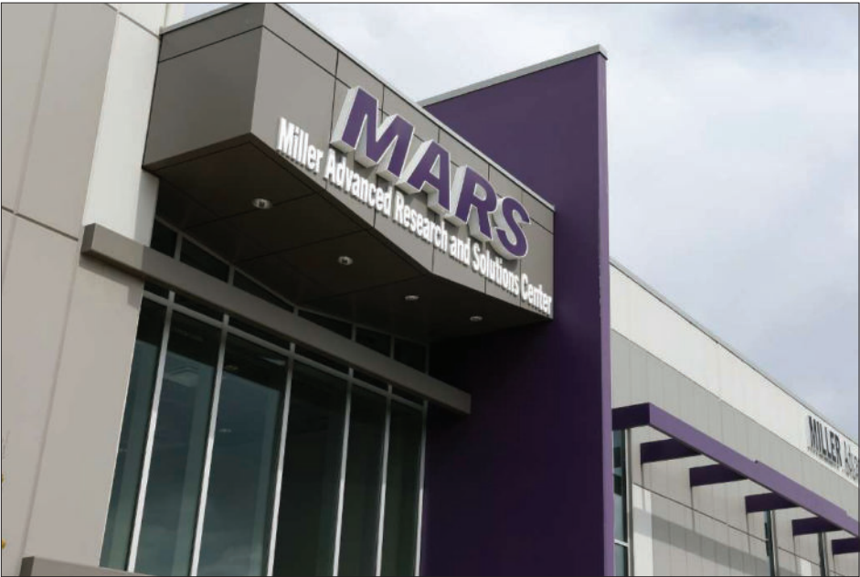
Photo courtesy of the Miller Advanced Research & Solutions Center.
