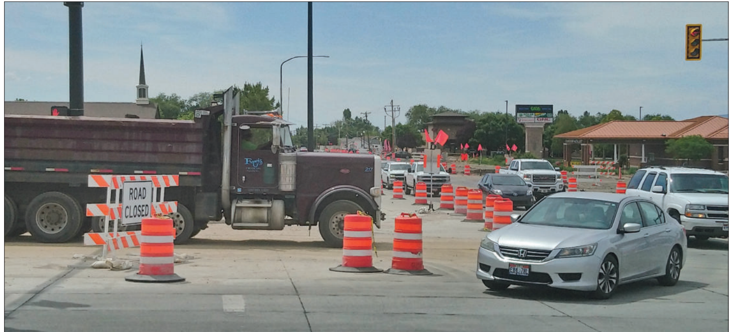
Traffic maneuvers through a road construction zone in Clinton. A recent assessment by a civil engineers association gave Utah roads a B-plus grade, the highest in the Utah infrastructure report card. (Brice Wallace/Salt Lake Business Journal)
