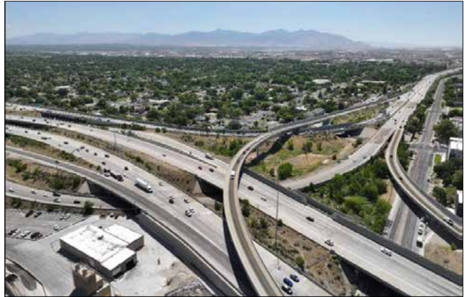
Highways snake through an area of Salt Lake City, with the Northwest Quadrant in the distance. The Utah Inland Port Authority and Salt Lake City are seeking public input as they develop plans for the best use of the area. (Photo courtesy Utah Inland Port Authority)
