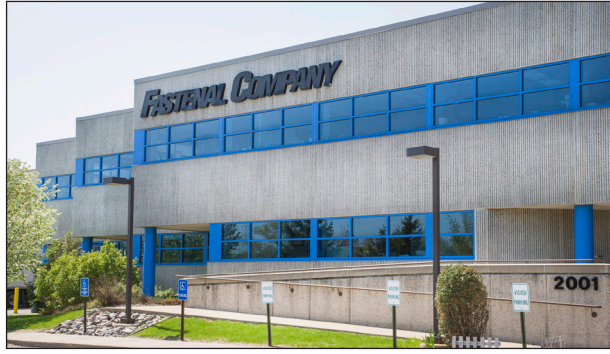
Global industrial products supplier Fastenal Co. has opened a new distribution center in Magna that will serve the company’s customers in the Intermountain West from Canada to Mexico. (Photo courtesy Fastenal Co.)
