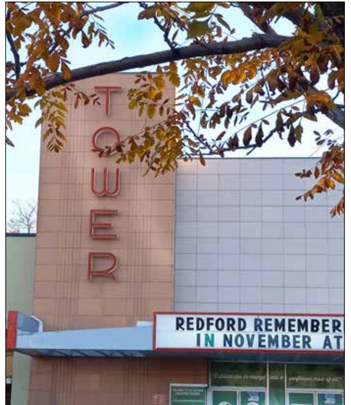
The historic Tower Theater sits vacant in Salt Lake City's busy 9th & 9th neighborhood on a recent Sunday evening. The very preliminary steps of a major restoration project have been taken with the Salt Lake Film Society's submission of drawings to city planners. (John Rogers, Salt Lake Business Journal)
