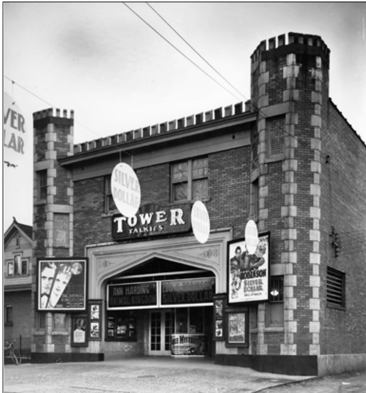
Posters advertising "The Animal Kingdom" starring Ann Harding and Edward G. Robinson in "Silver Dollar" adorn the Tower Theater — then called "Tower Talkies" — in 1932. The Salt Lake Film Society has taken preliminary steps in a major renovation of the landmark. (Photo from Cinema Treasures)
