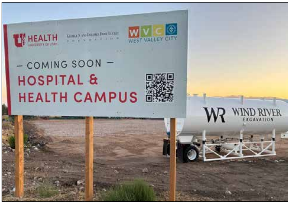
Construction of the University of Utah's new hospital starts in West Valley City. (Darrell Kirby/The City Journals)
