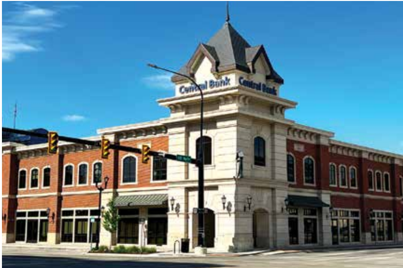
Central Bank Provo Office
