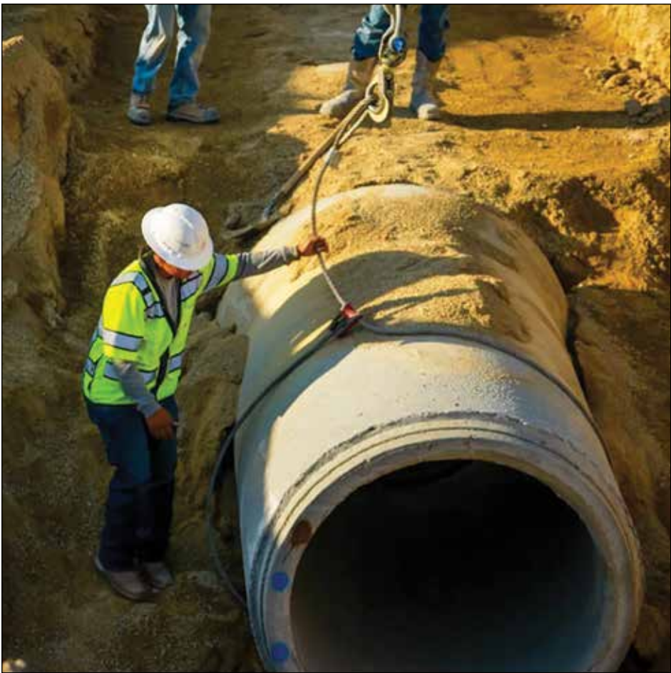
Drainage pipe was installed at The Point in Draper in 2025 as the project completed major infrastructure installation, including utilities, roads and site preparation. (Photo courtesy Point of the Mountain State Land Authority)
