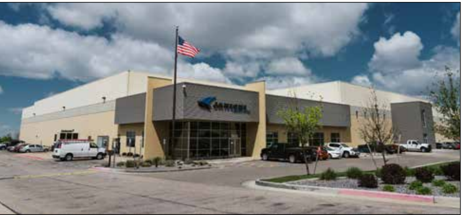
Janicki Industries’ 100,000-square-foot manufacturing site in Layton will receive a 70,000-square-foot expansion on the west side of the building. Construction will begin in June. (Courtesy Janicki Industries)
