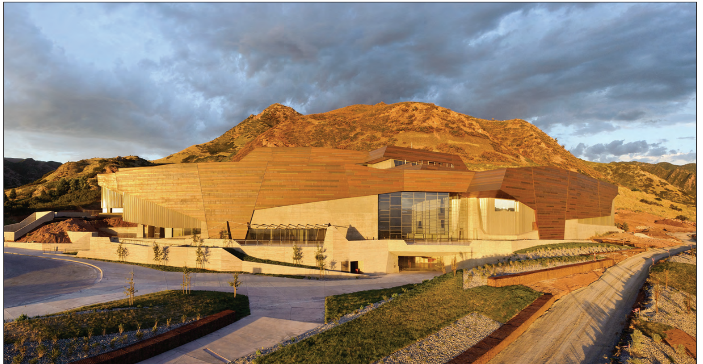
Both the parking structure and the non-landscaped portions of the roof at the new Utah Museum of Natural History make use of pervious concrete provided by Staker Parson.
