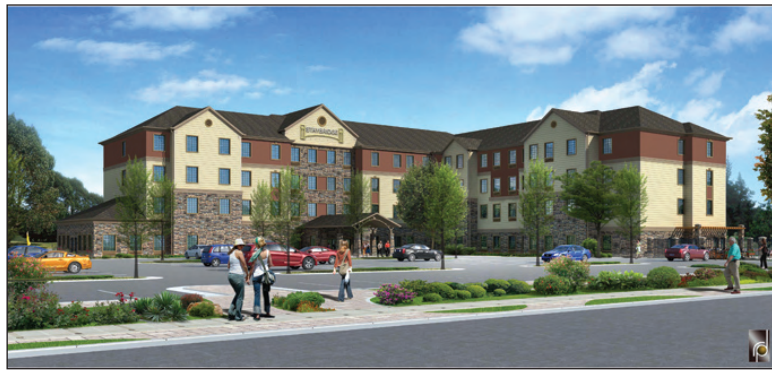
Artist's rendering of the Staybridge Suites hotel, which will be built within the View 20 Corporate Center in Midvale.
