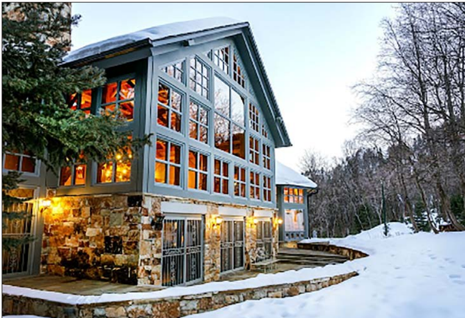
The Ashton lodge near Sundance Resort in Provo Canyon has been donated to Utah Valley University and will now house the Alan C. and Karen Ashton Center for Leadership and Inspiration for the university.
