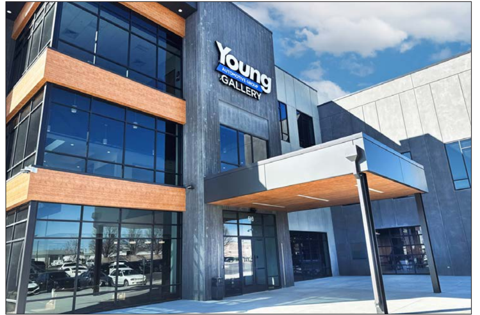
The Young Automotive Group has opened its new corporate headquarters in Layton. The company recently hosted a grand opening celebration for the 145,000-square-foot project with speeches from company executives and local government officials.
