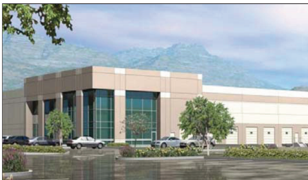
Bangerter Crossing Salt Lake City INDUSTRIAL
