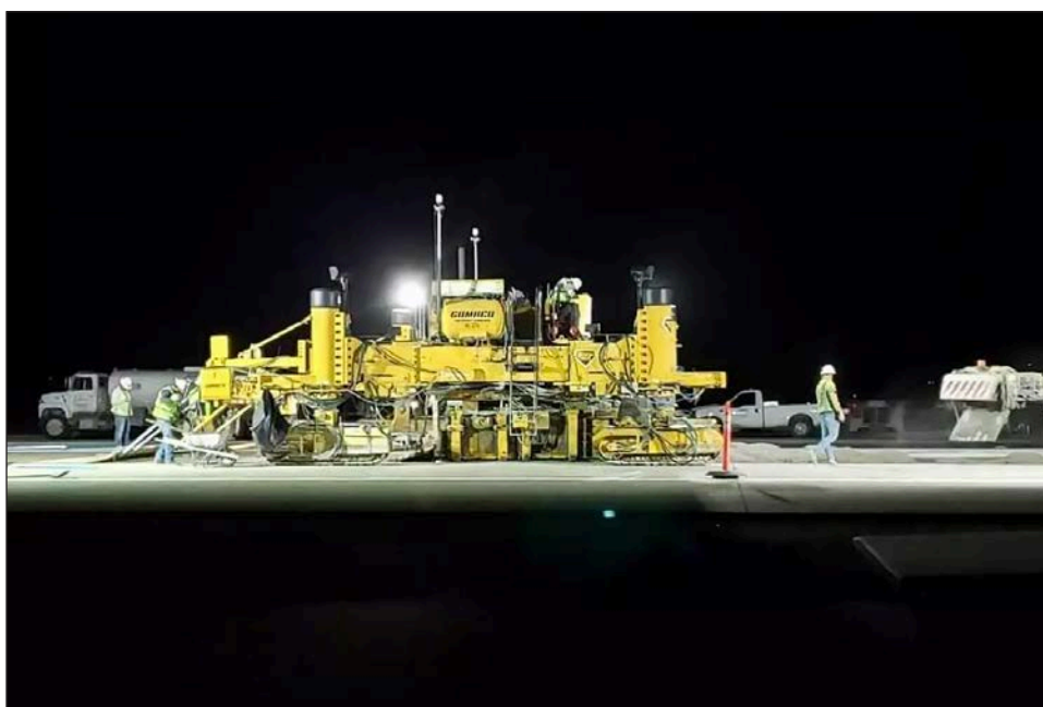
A crew from Murray-based Geneva Rock Products works on a runway repaving project at Hill Air Force Base in Northern Utah. Hundreds of Utah small businesses benefit from federal contracting projects throughout the state.
