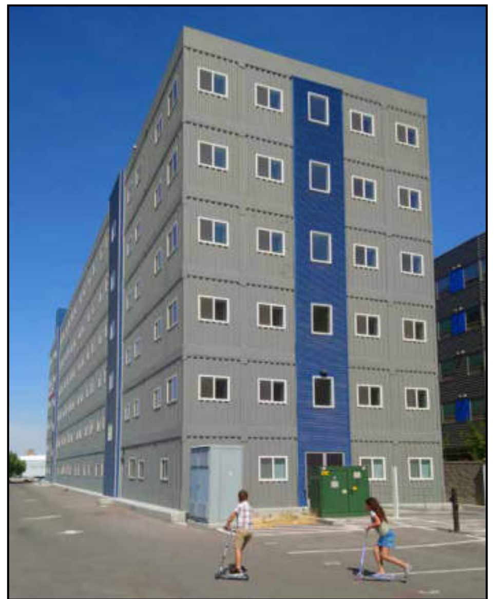
Children ride scooters around the back side of Box 500 Apartments in Salt Lake City. The six-stories apartment complex is an example of housing made from recycled shipping containers. (Brice Wallace/Salt Lake Business Journal)
