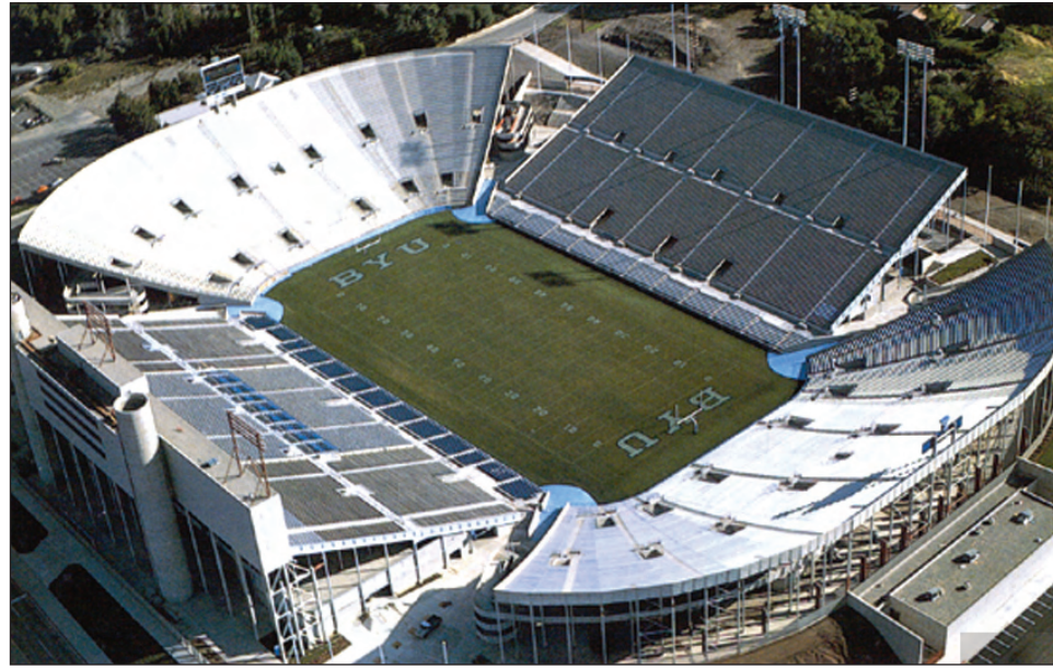
Layton completed a renovation and of expansion of Cougar Stadium at BYU in 1982.
