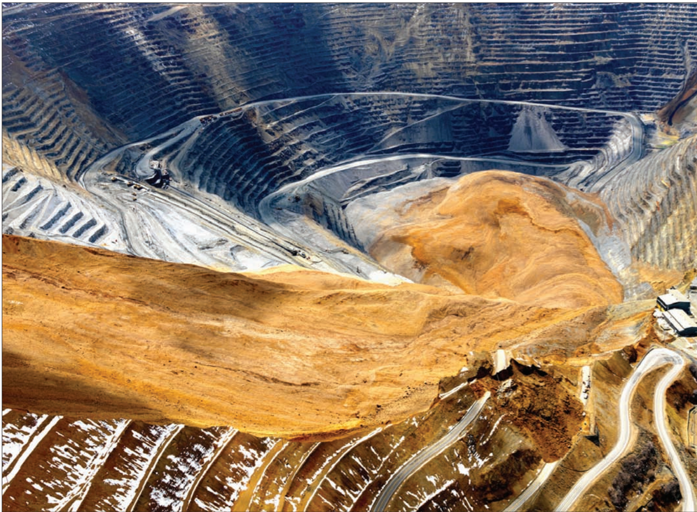
On April 10, 2013, 165 million tons of material broke loose from an upper region of Kennecott Utah Copper's mine in the Bingham Canyon of Salt Lake County. One year later progress is being made in restoring the mine to normal operation.
