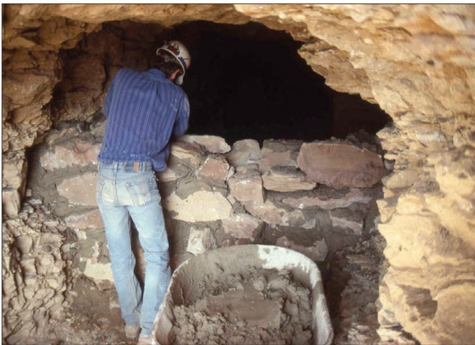
Most of the states where uranium mines are located have undertaken projects to seal the old mine entrances due to safety concerns. In recent months, mining speculators have begun opening the shafts and testing for the viability of renewed mining.
